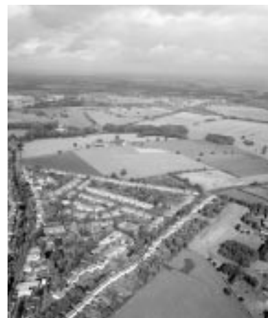
The stark boundary between the built up area and the green belt.
