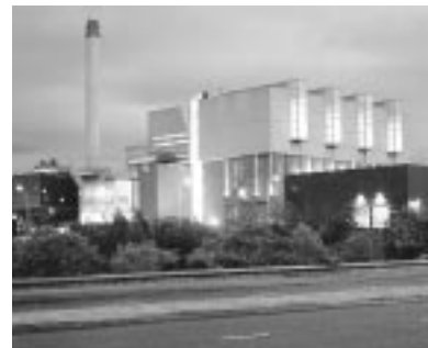
Tyseley Energy from Waste plant. 1
