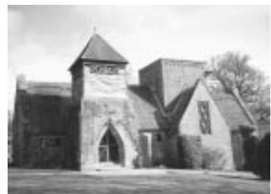
Brockhampton Church. A Grade I Listed Building.
