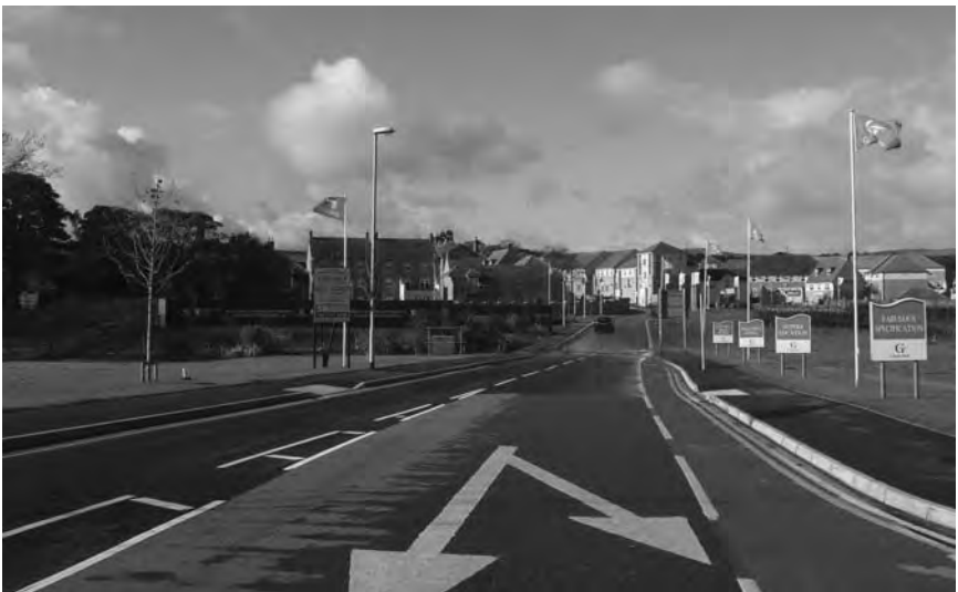
7.4 New development and access road, High Royds former psychiatric hospital site in Menston
